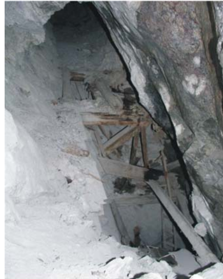
An Unacceptable Mine Test Site
