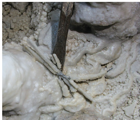
Figure 3: electrical cable remnants calcited into surfaces
