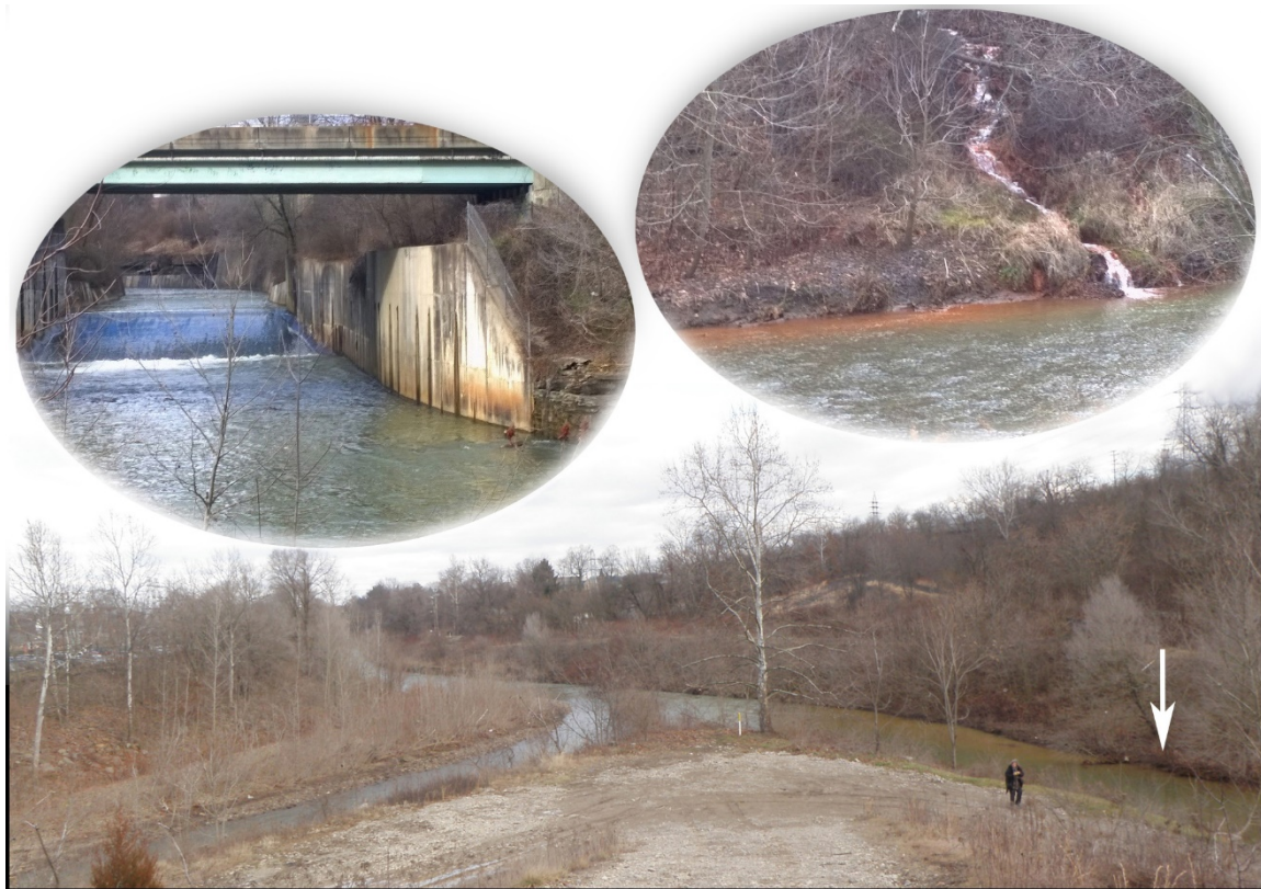
Figure 4: Bottom photo: confluence of the bypass channel (left) and back channel (right) of Chartiers Creek, looking downstream. Top left: dam on bypass channel, looking upstream. Top right: abandoned mine discharge (AMD) feeds into backchannel (arrow, bottom photo).
