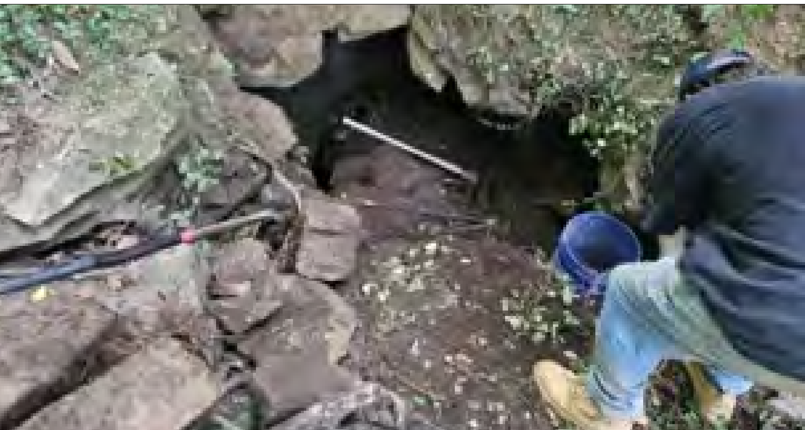
Shovels, a pickaxe, buckets, and PPE: Tools of the trade when trying to get back into the cave. Josh Farless is here, helping pull out some cinder blocks and boulders.
