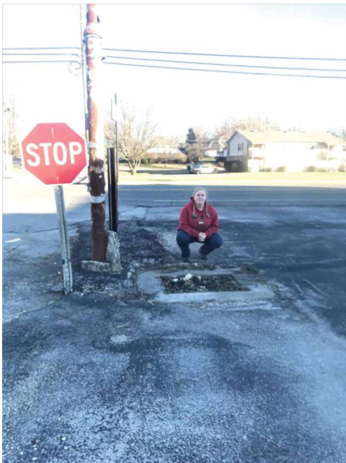
Figure 4. Horse Cave car wash storm drain.
