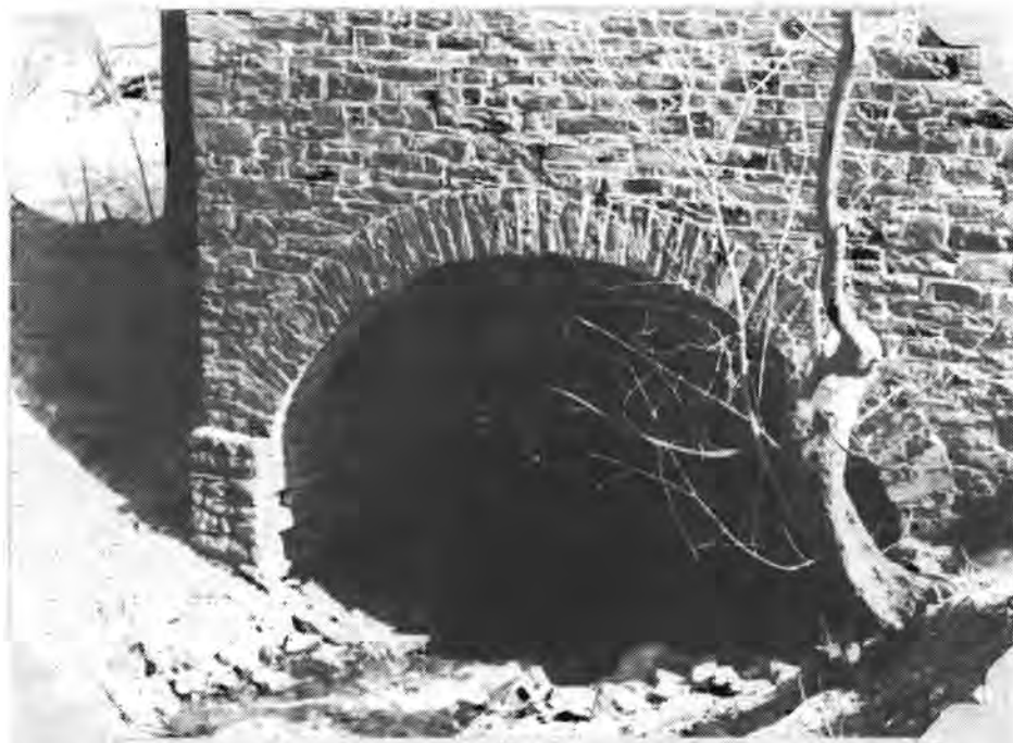
The archway above the millrace is unusual because it lacks a keystone.
