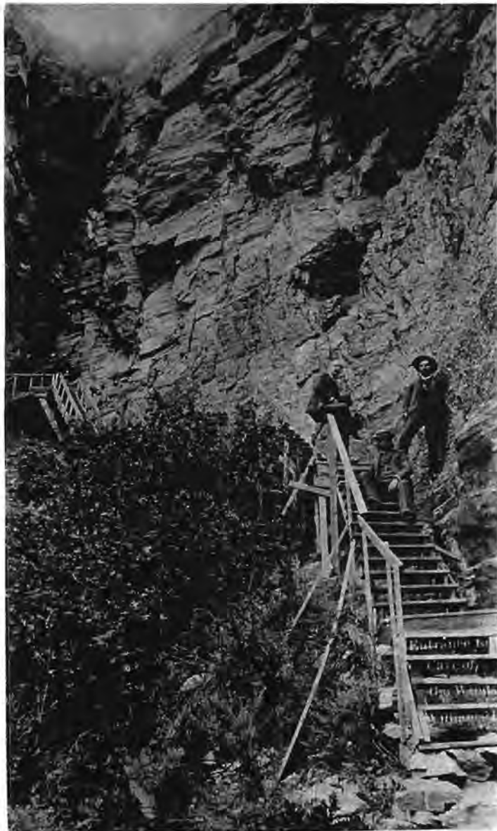
STAIRWAY TO ORIGINAL ENTRANCE OF CAVE OF THE WINDS
