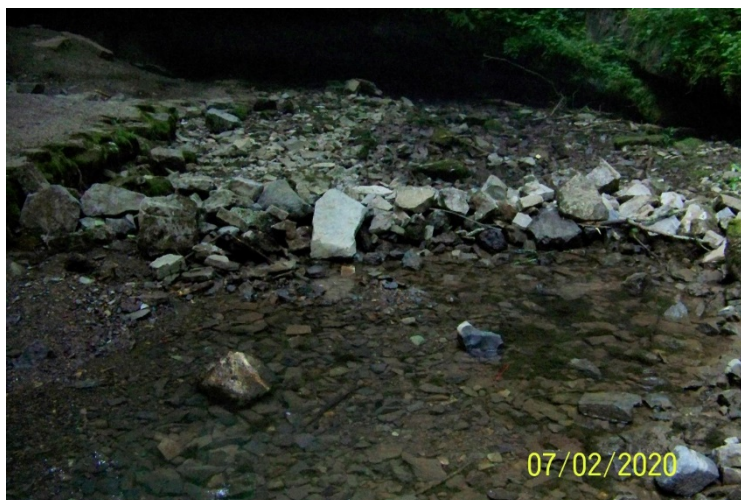
Damn placed illegally at Tytoona Preserve
