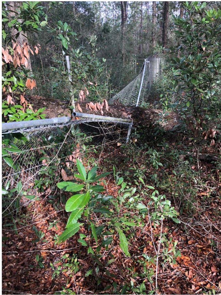
Fence damage from a fallen snag (Photo by Lori Hempfling)
